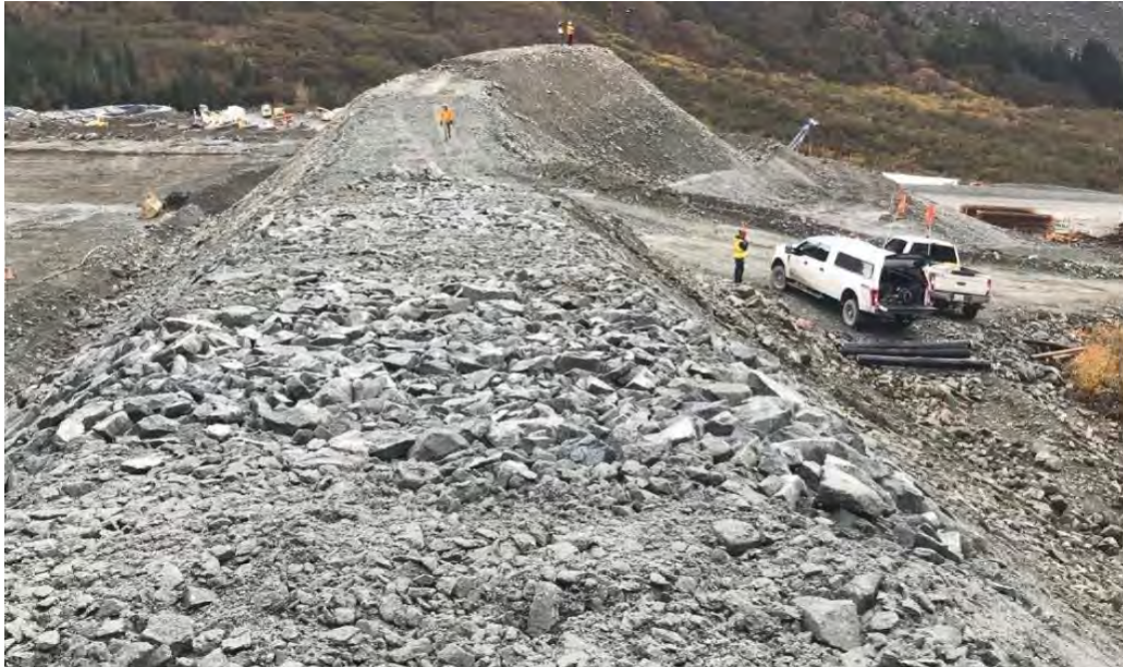
Figure 4-3: Avalanche diversion berm constructed with onsite cut-fill loose rock material with upslope and downslope angles at approximately 34° (photo Ross and Johnson, 2019).
